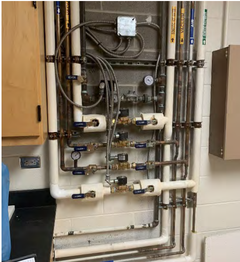
Laboratory Manifold
