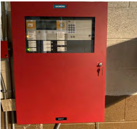
Fire Alarm Control Panel
