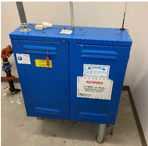
Elevator Controller / Hydraulic Pump
