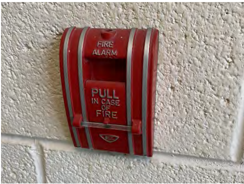
Fire Alarm Pull – Not ADA Height
