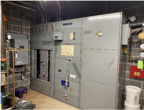
Electrical Power System MDP
