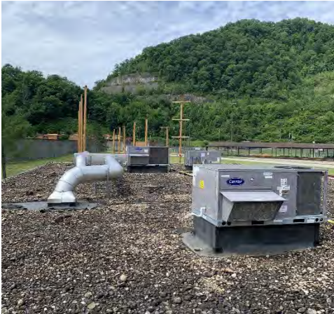
Rooftop HVAC Units and Ductwork
