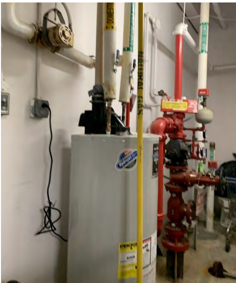
Water Heater / Sprinkler System Entrance
