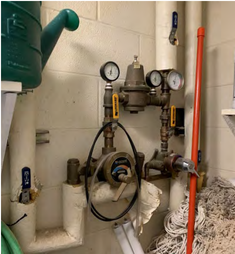
Thermostatic Mixing Valve
