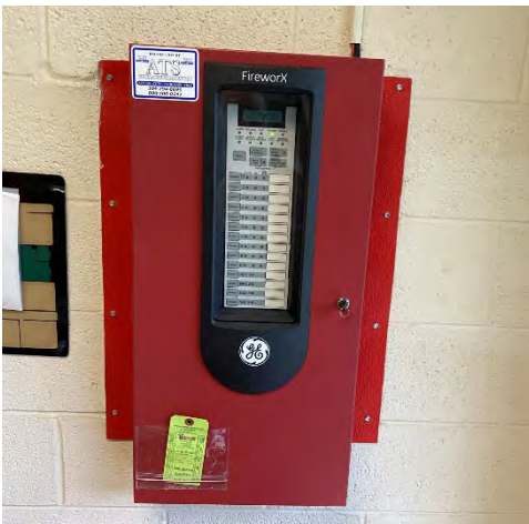
Fire Alarm Control Panel
