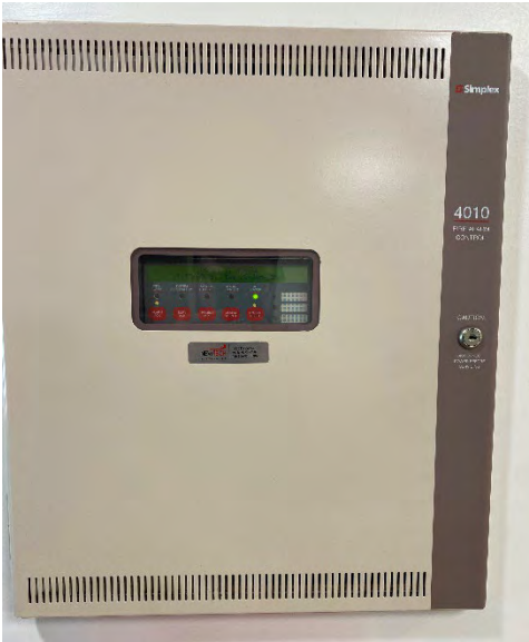
Fire Alarm Control Panel
